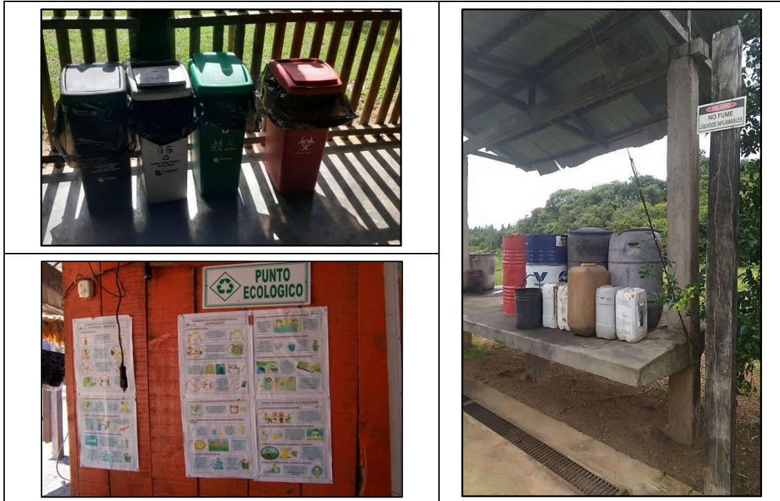
Image 11. Signs used in the projects for proper waste management and disposal. The oil and fuel handling areas are isolated and have channels for collection in case of any type of spill.
